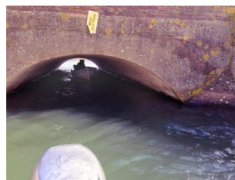
Limited headroom through the causeway tunnel
